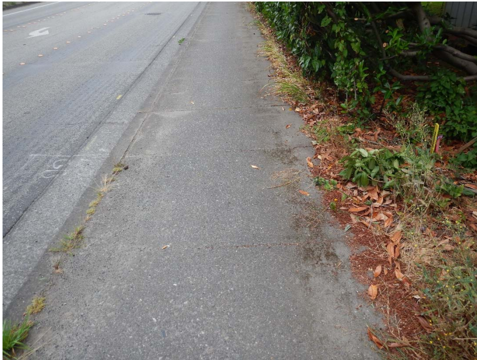
Photo 3. View north on Yew Street of northwest property corner, sidewalk, curb, and gutter.
