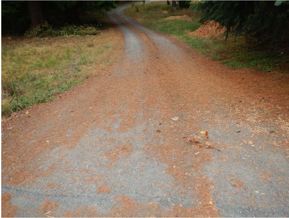
Photo 1. View east of the existing driveway at 1204 Yew Street.
