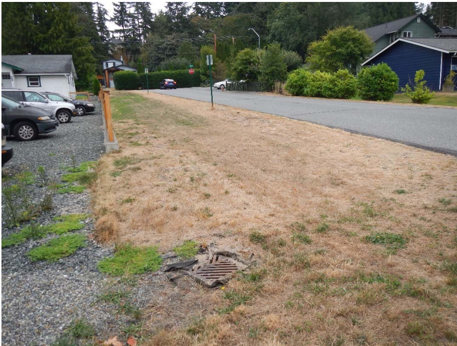
Photo 6. View east on Old Lakeway Dr. from third grate.
